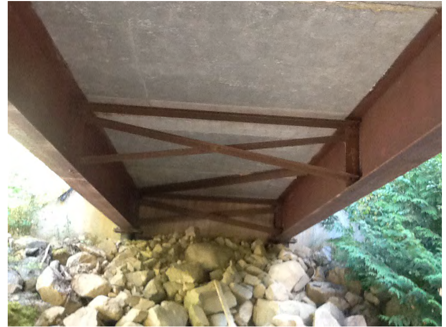
Underside of bridge
