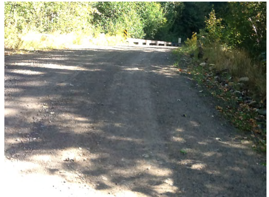
Right approach facing structure
