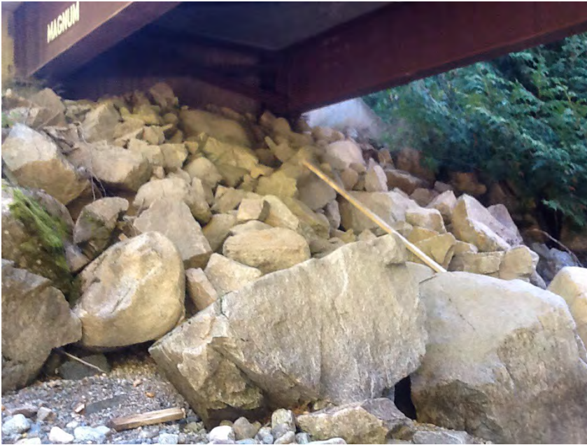
Left Bank Abutment when facing downstream
