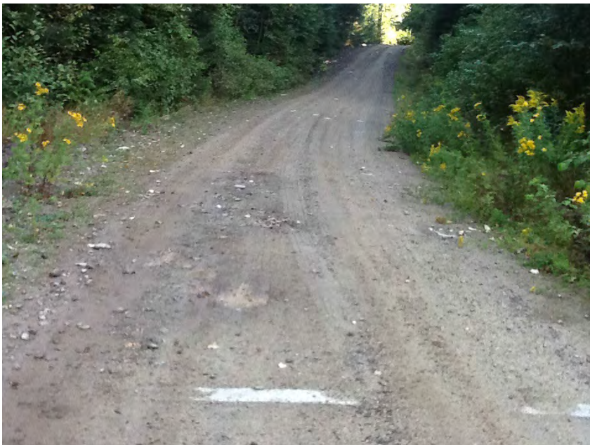
Left approach facing away from structure
