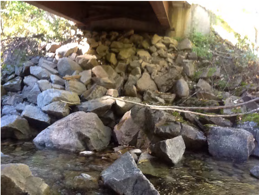
Right Bank Abutment when facing downstream
